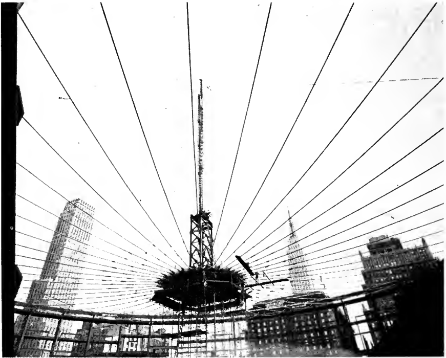
The tension ring and the erection derrick rested on a tubular scaffolding tower, which was set on a system of temporary timber cribbing on the arena floor. The forty-eight 3 \frac{3}{4} -in. diameter roof cables are ready to receive roof steel.
